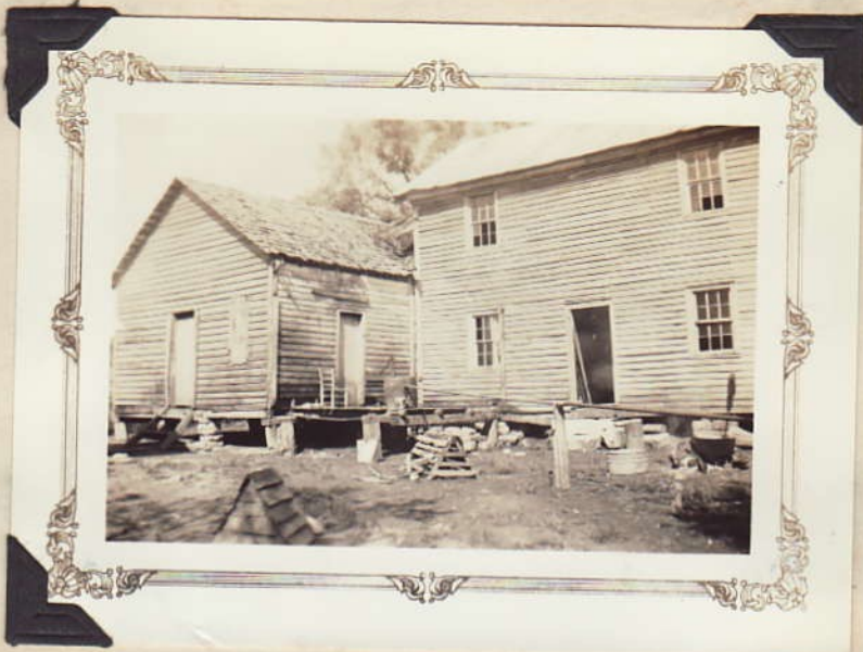
Rear View of William Davis Home
